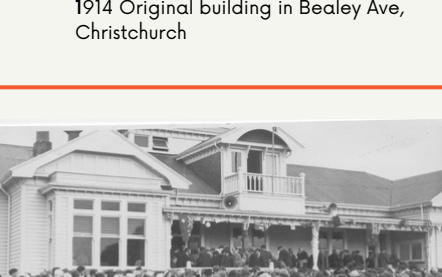
1914 Original building in Bealey Ave, Christchurch
